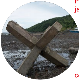
A concrete jackstone, part of an artificial reef.
