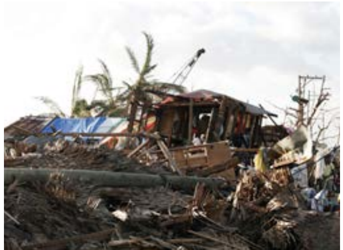
This home in the Philippines was destroyed by Typhoon Haiyan in November 2013.
